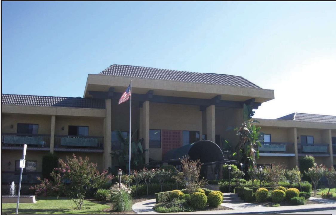
Adjacent convalescent home/retirement facility to the north at 720 W. Camino Real Ave – Building frontage along W. Camino Real Ave
